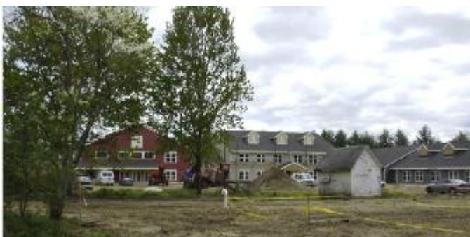
Photo taken during construction, circa 2001.
