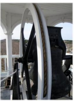
the top. The curved yolk extends down toward the middle of the bell where it is attached to two round axle-like poles on each side that rest on the cradle frame. The bell rope is secured to a huge wheel which turns when the rope is pulled, turning the wheel axles and swinging the bell. The clapper is hooked to the inside of the bell at the top and swings independently. When the bell swings, the clapper hits one side of the bell and then the other making the ding-dong sound.
