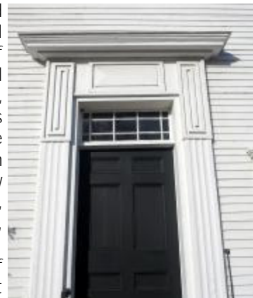
One of three front doors to the church showing the molding.
